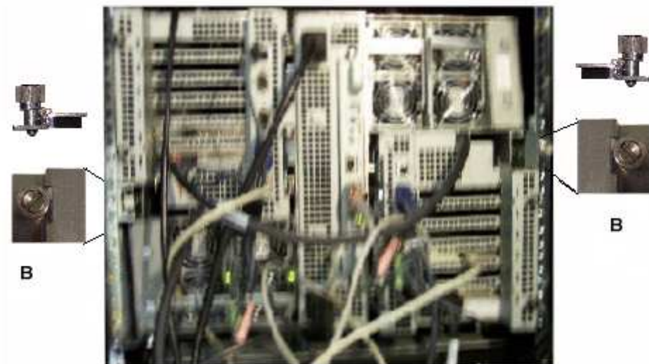
Figure 5. Installing rear stoppers.
