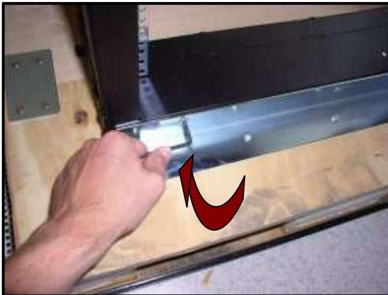
Figure 13. Removing shipping brackets
