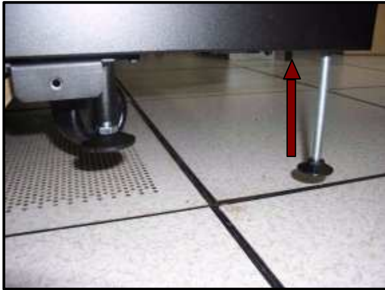
Figure 23. Installing the rear jack screws
