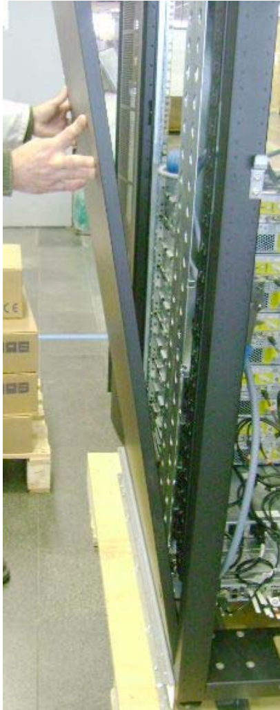
Figure 20. Installing a side panel
