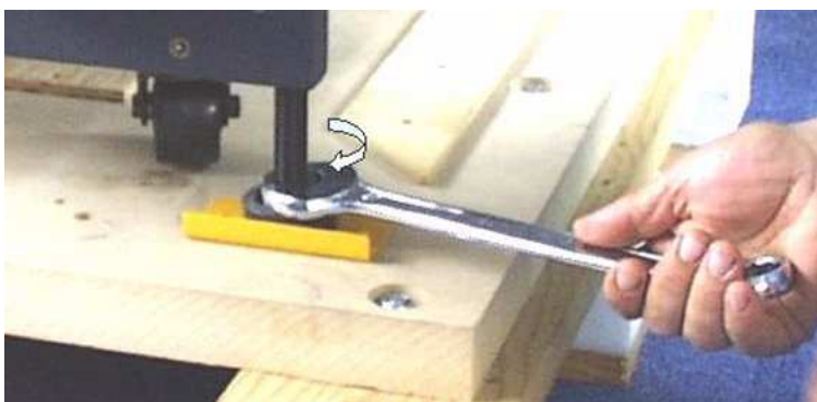
Figure 10. Lowering cabinet jacking screws – 36U cabinet
