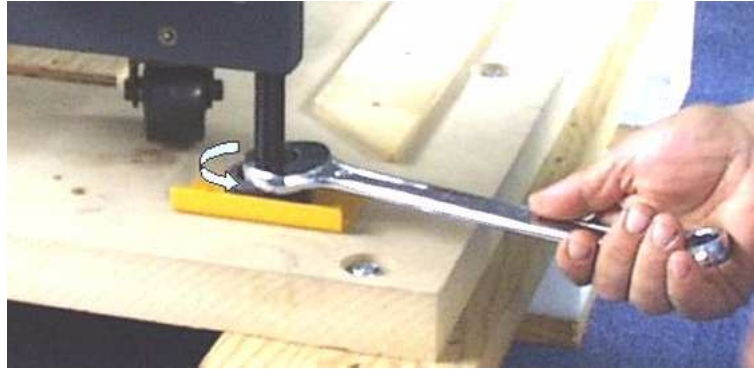
Figure 13. Cabinet jacking screws and retaining brackets – 36U cabinet
