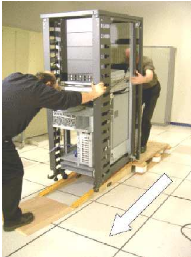
Figure 14. Unloading the 36U cabinet
