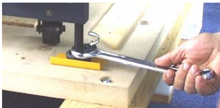
Figure 10. Lowering cabinet jacking screws – 36U cabinet
