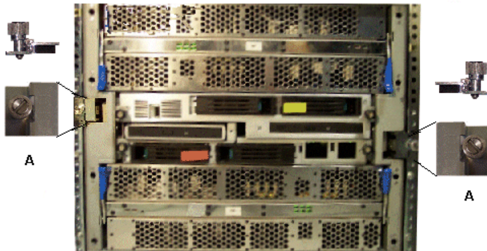
Figure 4. Installing front stoppers
