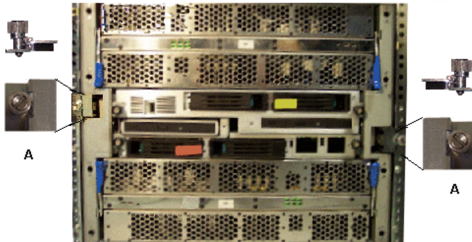
Figure 4. Installing front stoppers
