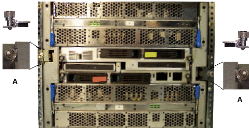
Figure 4. Installing front stoppers
