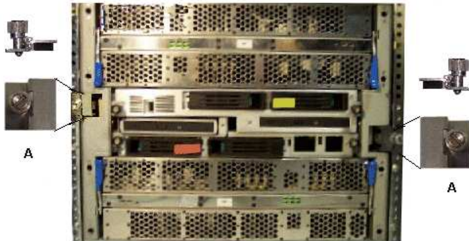
Figure 4. Installing front stoppers
